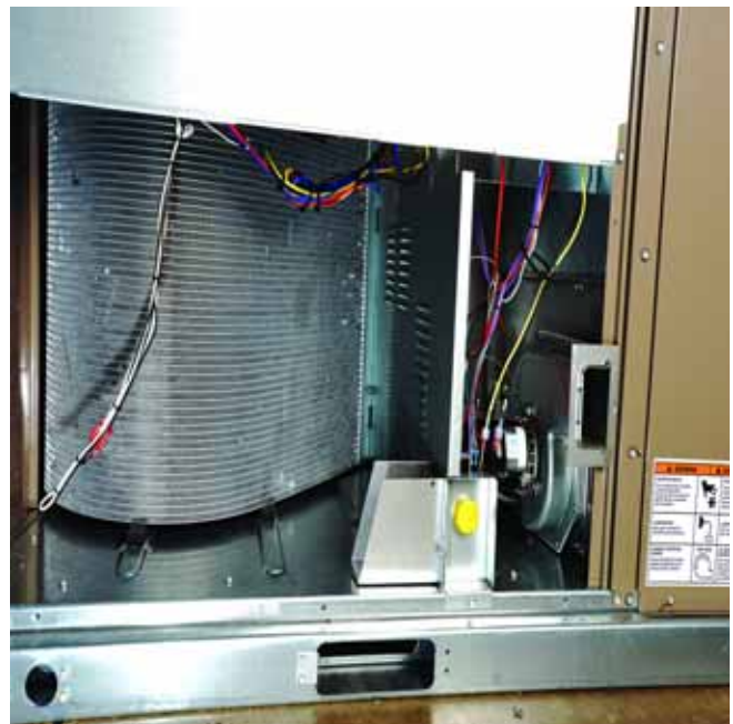
Figure 16: Flue Exhaust Hood Shipping Location
